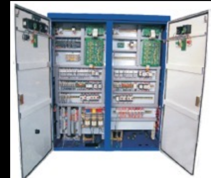
Main control panel with double side access to all components
